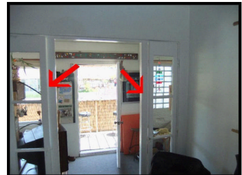
NON-TEMPERED GLASS - SIDE LIGHT WINDOWS
