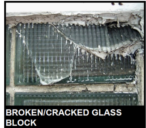
GROUT DETERIORATED/MISSING
