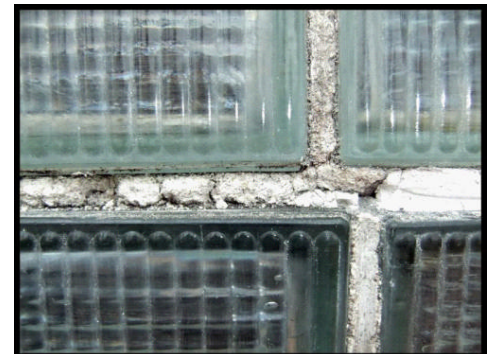
GROUT DETERIORATED/MISSING
